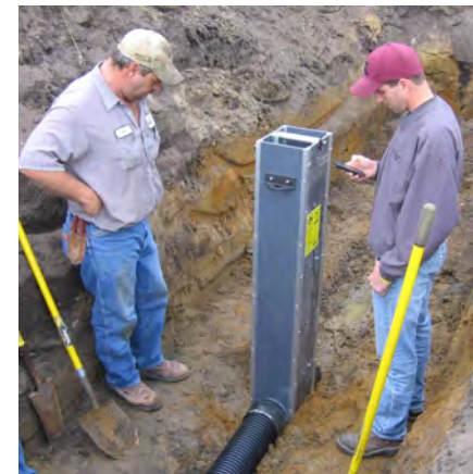
Stop Log Structure
